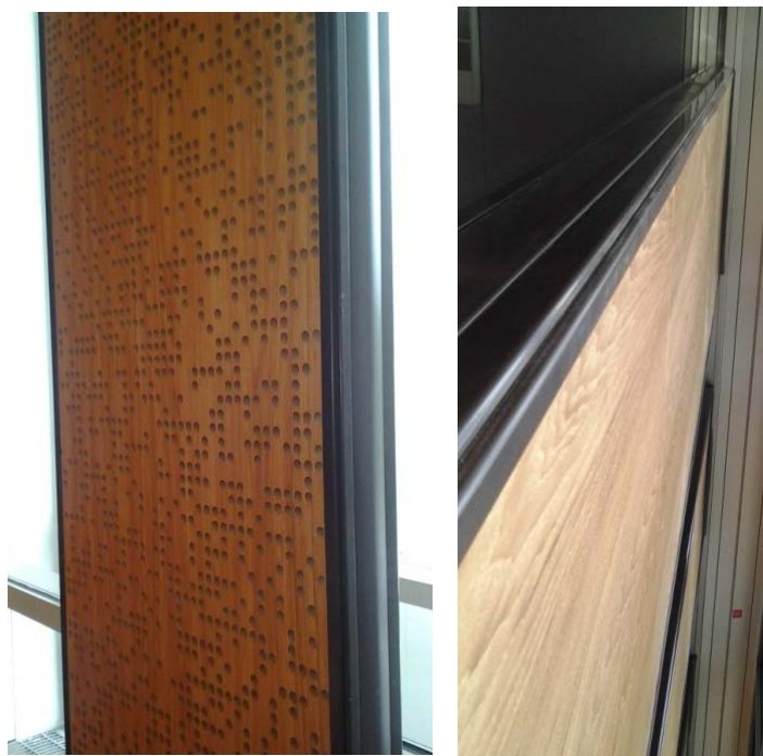
Figure 4.4 Variable acoustic panels in the Tracking Room – absorptive side (left); reflective side (right)
