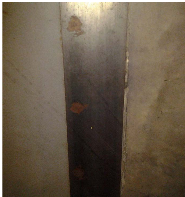
Figure 5.5- Junction of isolated and fixed slabs bridged by sheet metal.
