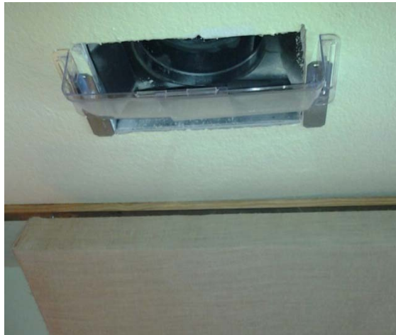
Figure 3.9- HVAC diffusers were removed throughout the studio.
