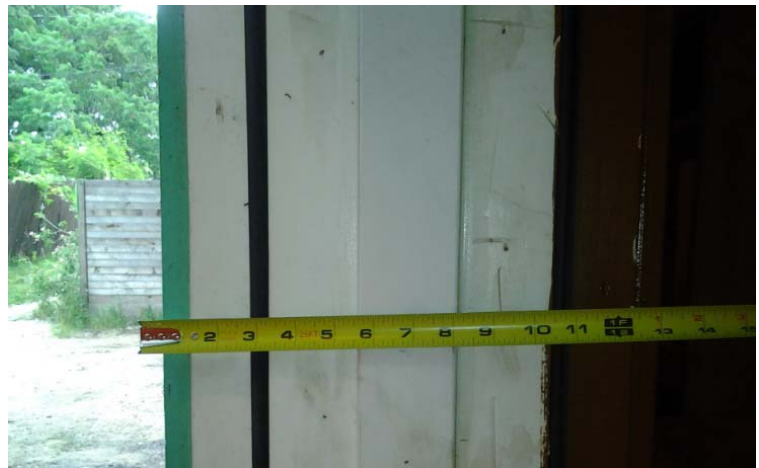
Figure 3.4- Exterior wall is more than 12" thick.
